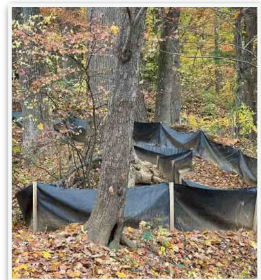
Trail Erosion Control
