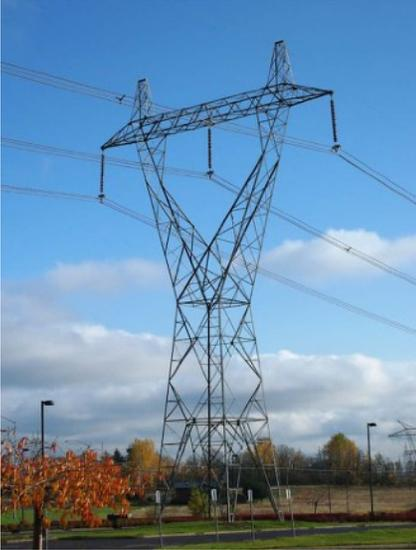
High voltage, long range power transmission line metal support structure.
